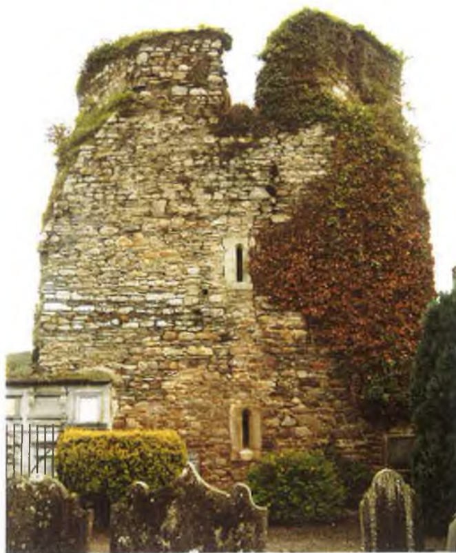
FIG. 6.44 Octagonal tower at Augustinian priory, Inistioge (Co. Kilkenny).
