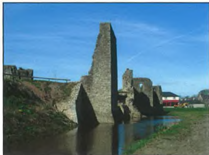
FIG. 6.23 Tower 2 viewed from southeast
