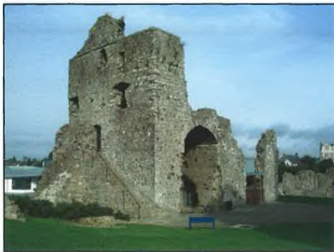
FIG. 6.26 West gatehouse viewed from south.
