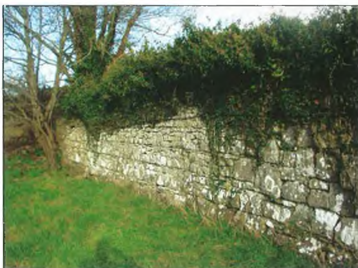
FIG. 5.10 Part of the 80m section of wall surviving in the grounds of Crowpark House. The large stones and style of block-work to the right suggest medieval construction. (February 2002).
