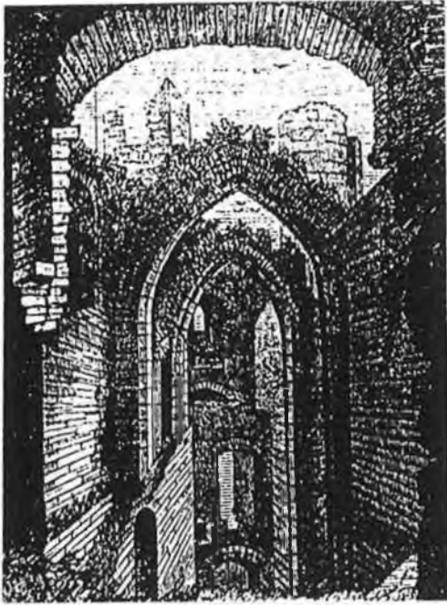
FIG. 6.19 Nineteenth-century drawing showing third floor of keep divided and arches spanning third floor of hall. Source: Dub. Penny Jn. , ii, no. 44 (1833), p. 253.
