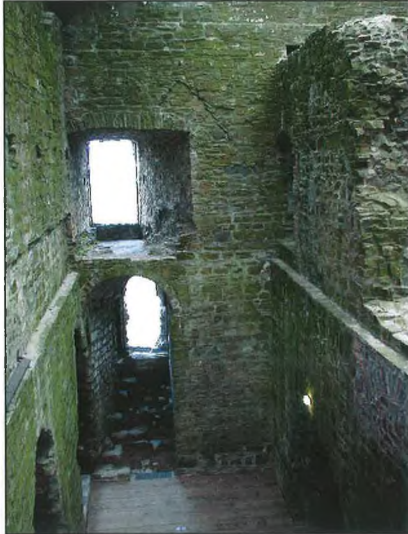
FIG. 6.18 Second floor of chamber viewed from south.
