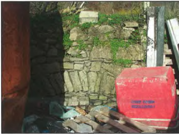
FIG. 5.5 The remains of a neatly built (but now blocked up) arch can be seen 2m east of the site of the southwest corner tower (February 2002).
