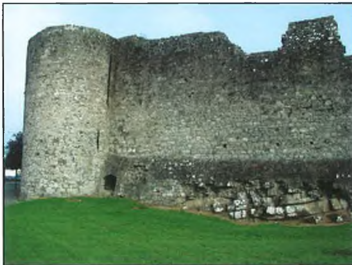
FIG. 6.29 Tower B, sallyport and section of curtain wall, viewed from southwest. Note bedrock behind robbed out base-batter.
