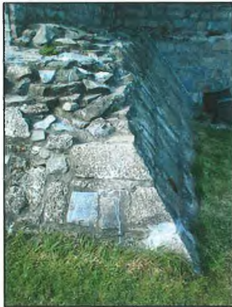
FIG. 6.22 The corner stones of the plinth.
