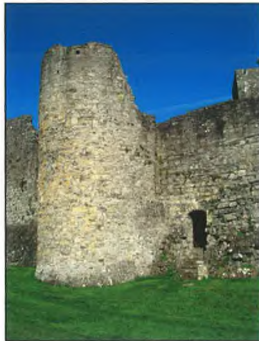
FIG. 6.30 Tower C and sallyport, viewed from south.
