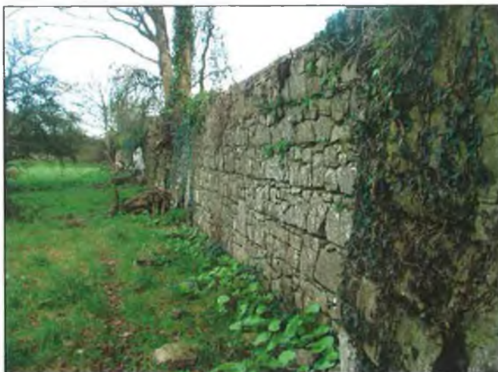
FIG. 5.9 West façade of west wall, viewed from southwest. One of the finest surviving stretches of the town wall at Trim is in the grounds of Crowpark House. The style of block-work in this section suggests post-medieval reconstruction. This would tie in with seventeenth-century recommendations that repairs be carried out on the wall. Note the trees growing on the wall! (February 2002).
