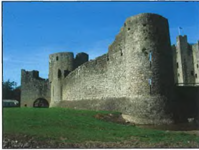
FIG. 6.36 Barbican Gate, curtain wall and Tower E, viewed from east.
