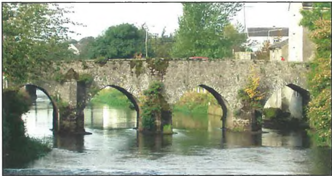
FIG. 5.20 The old bridge at Trim, viewed from downriver (east side)
