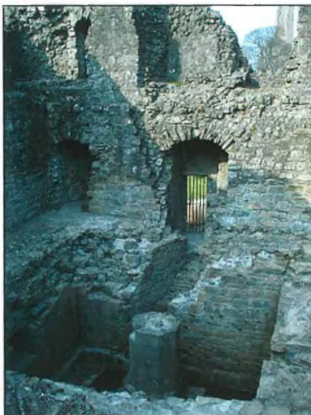
FIG. 6.40 Interior of solar (Tower 3), viewed from south. Note inserted octagonal pillar in basement.
