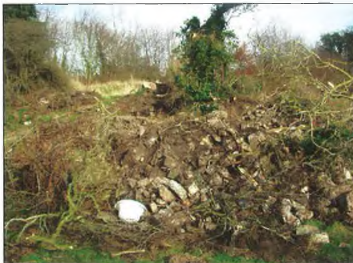
FIG. 5.8 Along the west side of the town, south of the Boyne, the removal of trees in advance of property development has resulted in irreparable damage to at least one segment of wall (February 2002).
