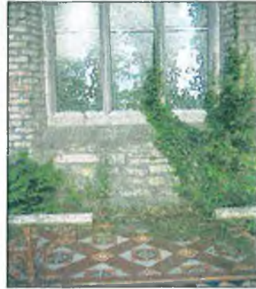
E chancel with rails and floor tiling still intact.
