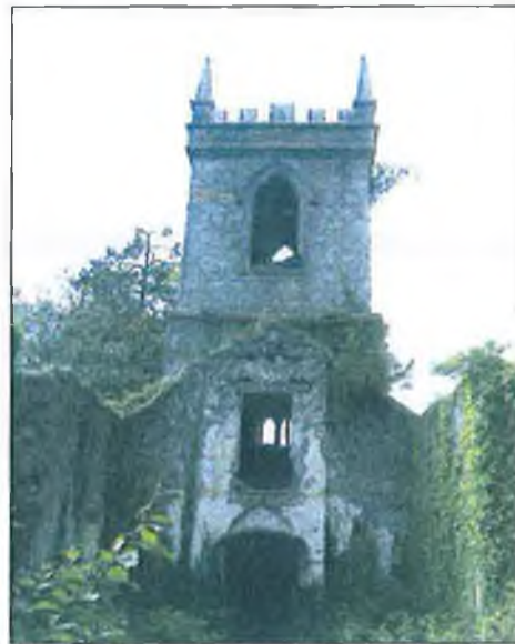
E chancel to W tower
