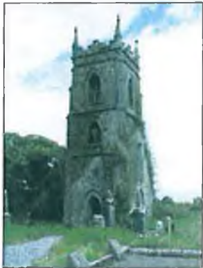
Tower at SE
