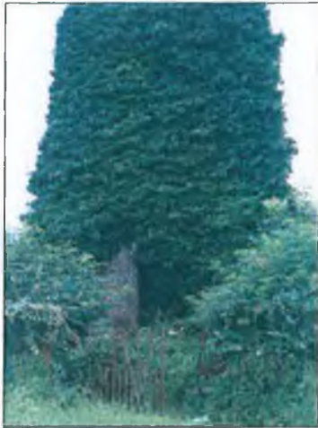
Remains of W tower
