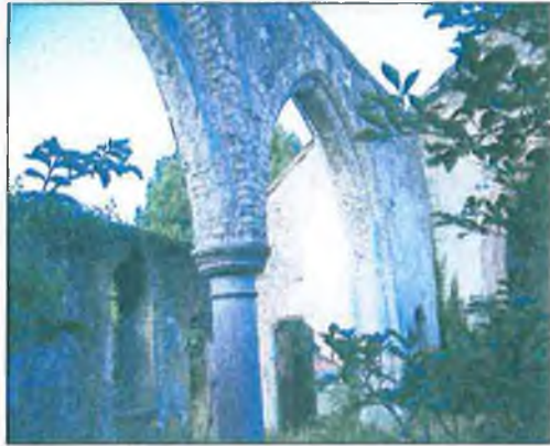
N aisle and vestry entrance from W
