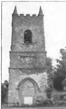
SW tower face
